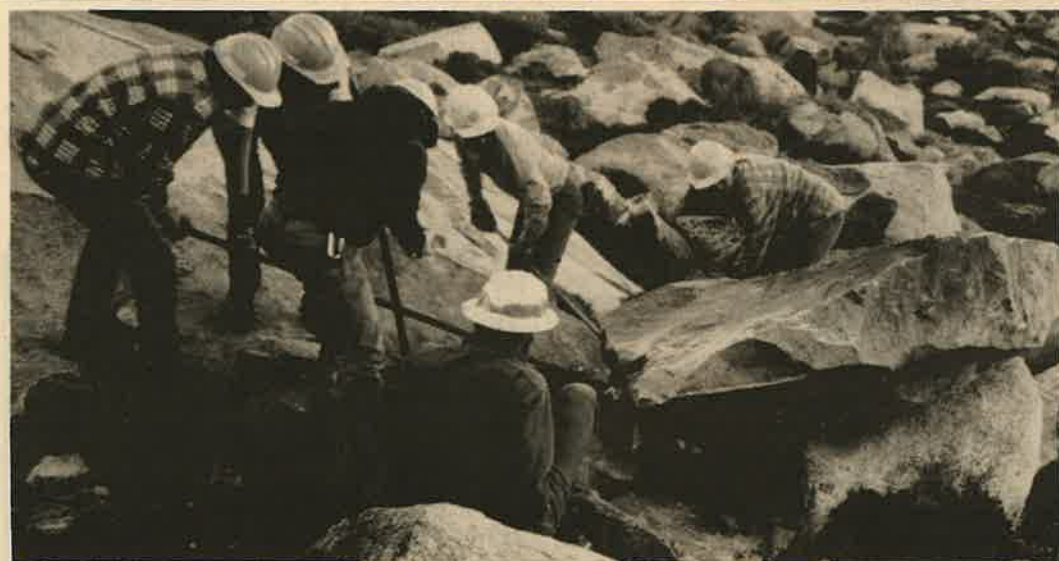
Boulders weighing up to 3 tons were moved during work on the Post Peak Pass Trail re-route; a total of over 180 tons of material were moved by hand over the course of the 1989 summer. U.S. F.S. photo
